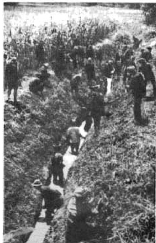
building irrigation systems.
